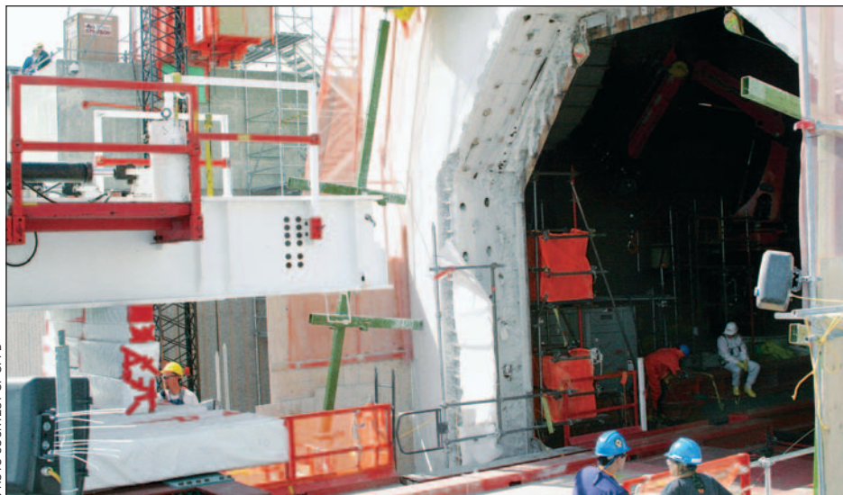
Fort Calhoun workers cut a large hole in the 4-foot-thick containment building to replace the vessel head.
