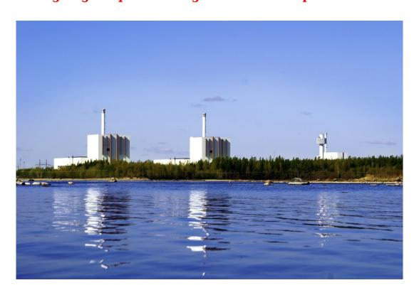
The electricity output from a nuclear power plant varies even when the reactor itself is operating at constant power. The turbine efficiency is dependent on the sea water temperature. The turbine is more efficient when cooled with really cold water, therefore the electricity production is the highest in the winter even though the reactor produces the same amount of energy all year round.
